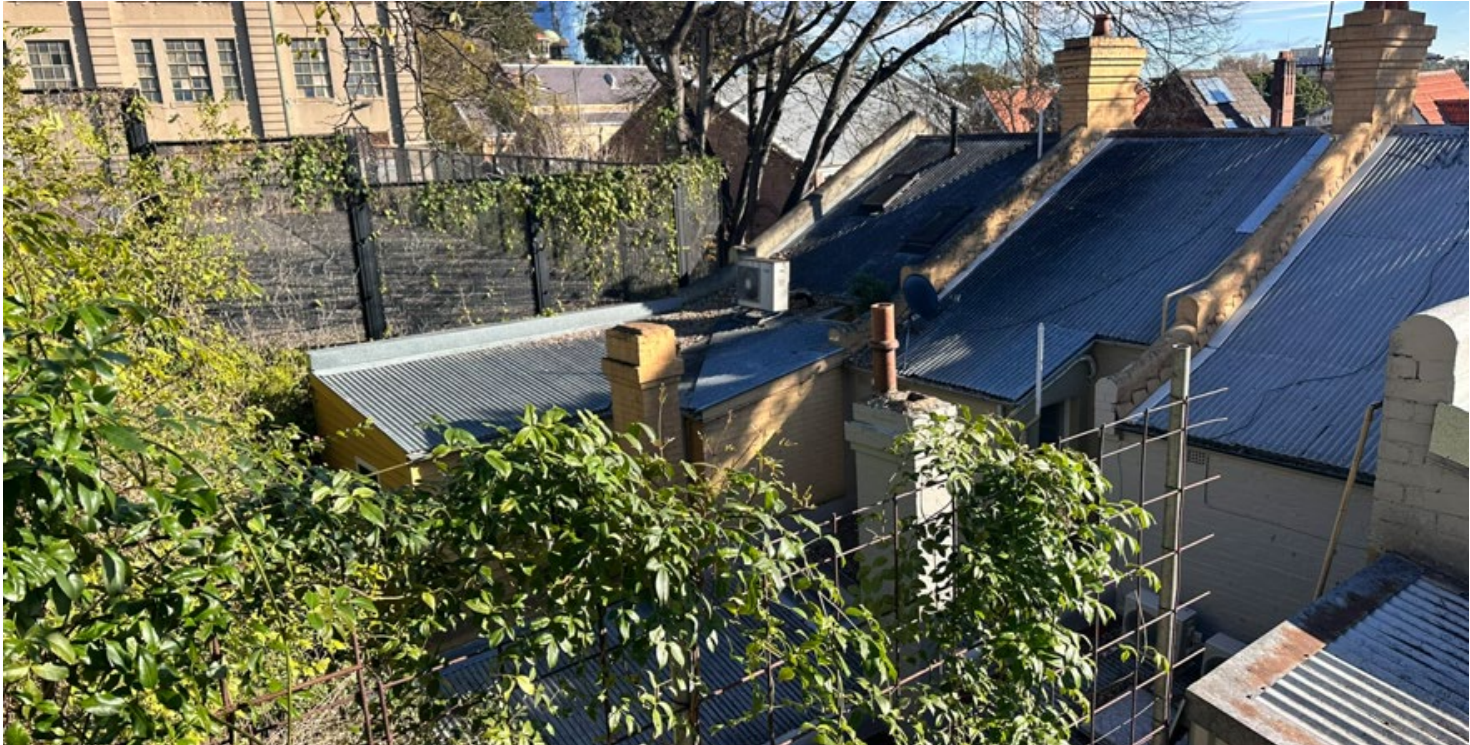
view to the rear of 18 and 22 Trinity Avenue
