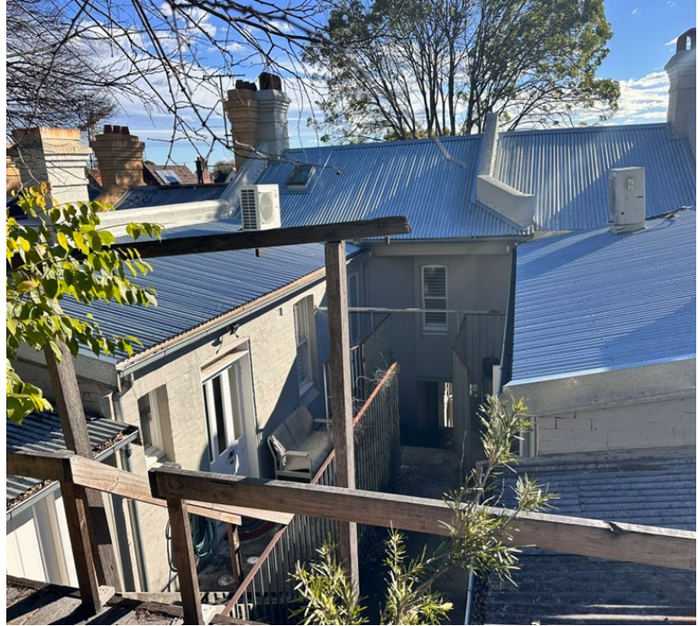
Rear elevation, looking west
